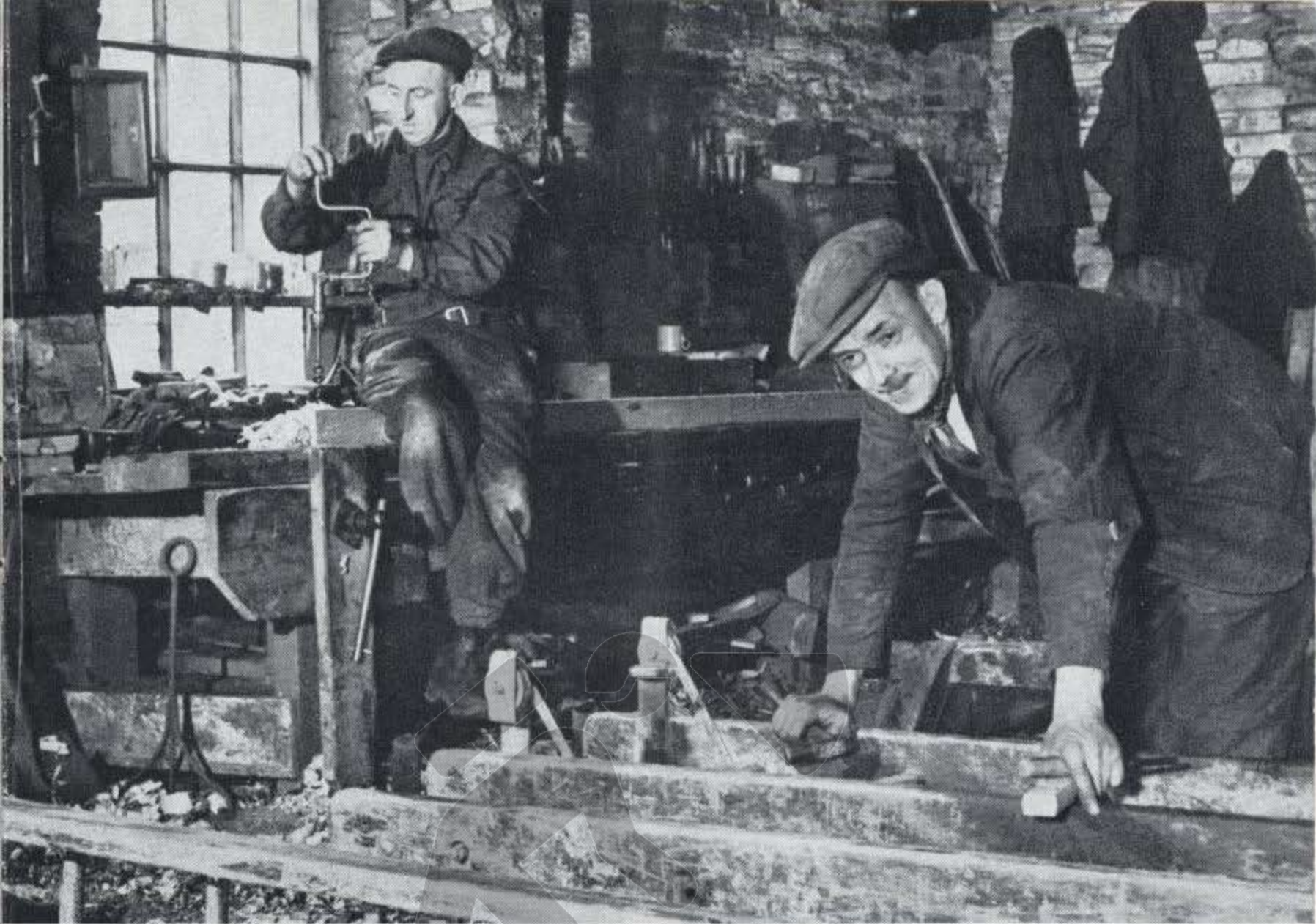
The Carpenters' Shop
