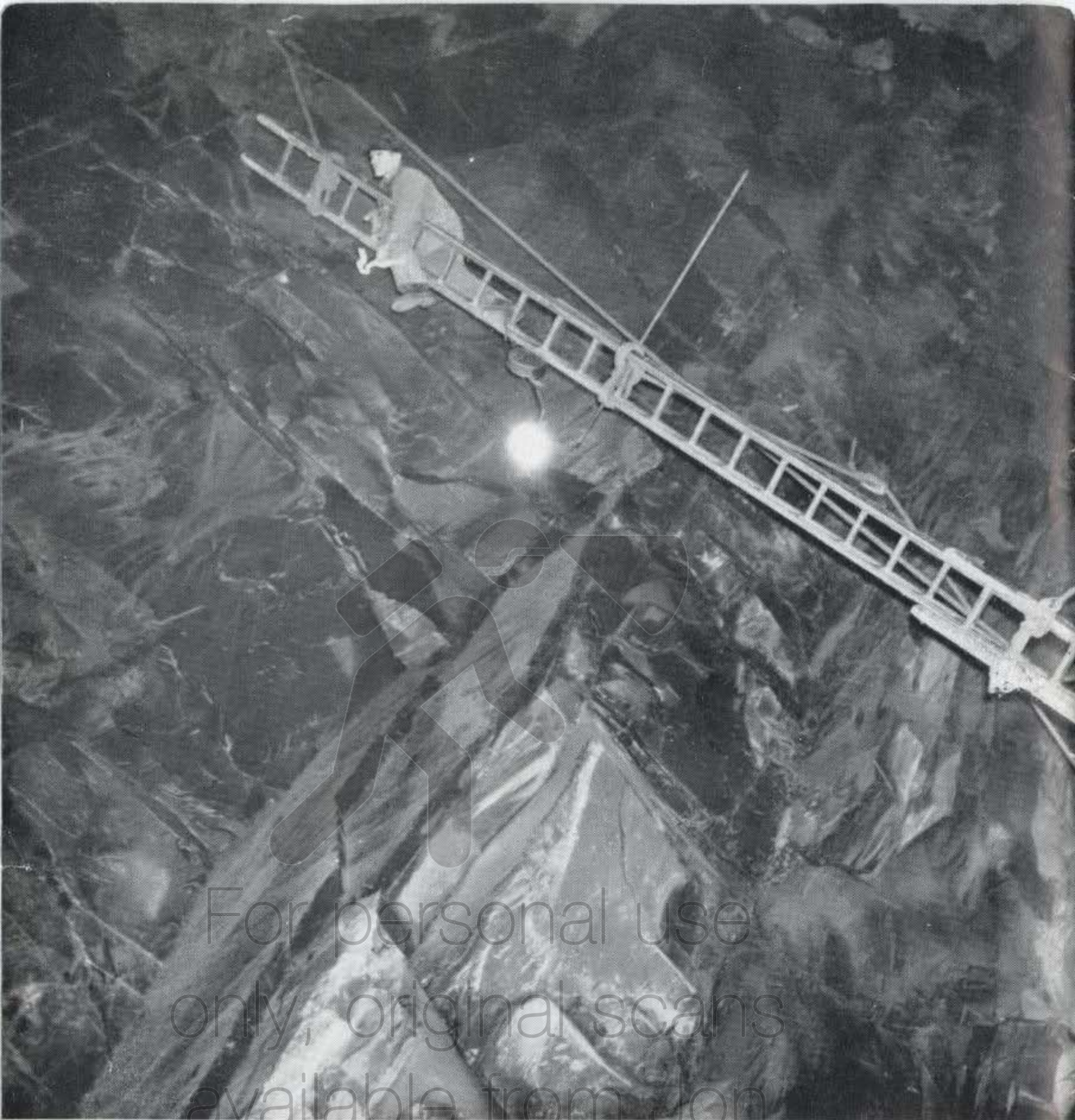
LIKE MASONS IN A CATHEDRAL—the securers work on the roof of a chamber at Oakeley, to remove any loose rock which might endanger those far below.
