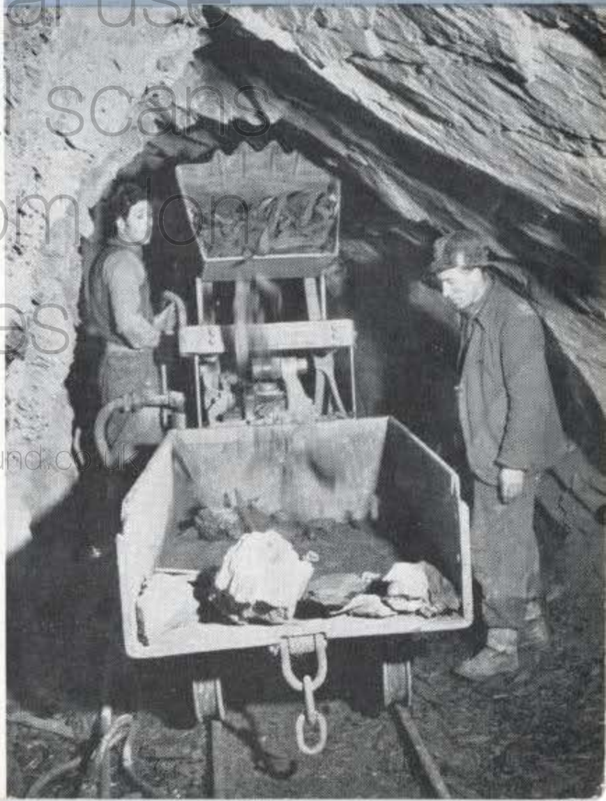
(Below.)—Machines such as the EIMCO mechanical shovel speed the routine tasks.
