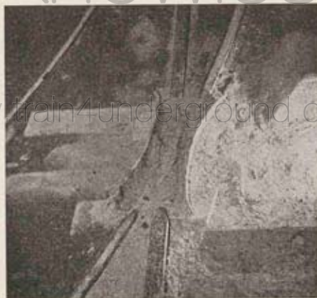
"Platan groes" — Flat plate used to cross from one tram-road to another.
