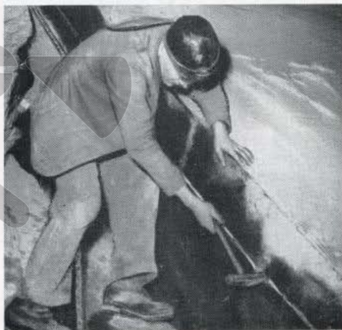
Hammering the "plug and feathers"
