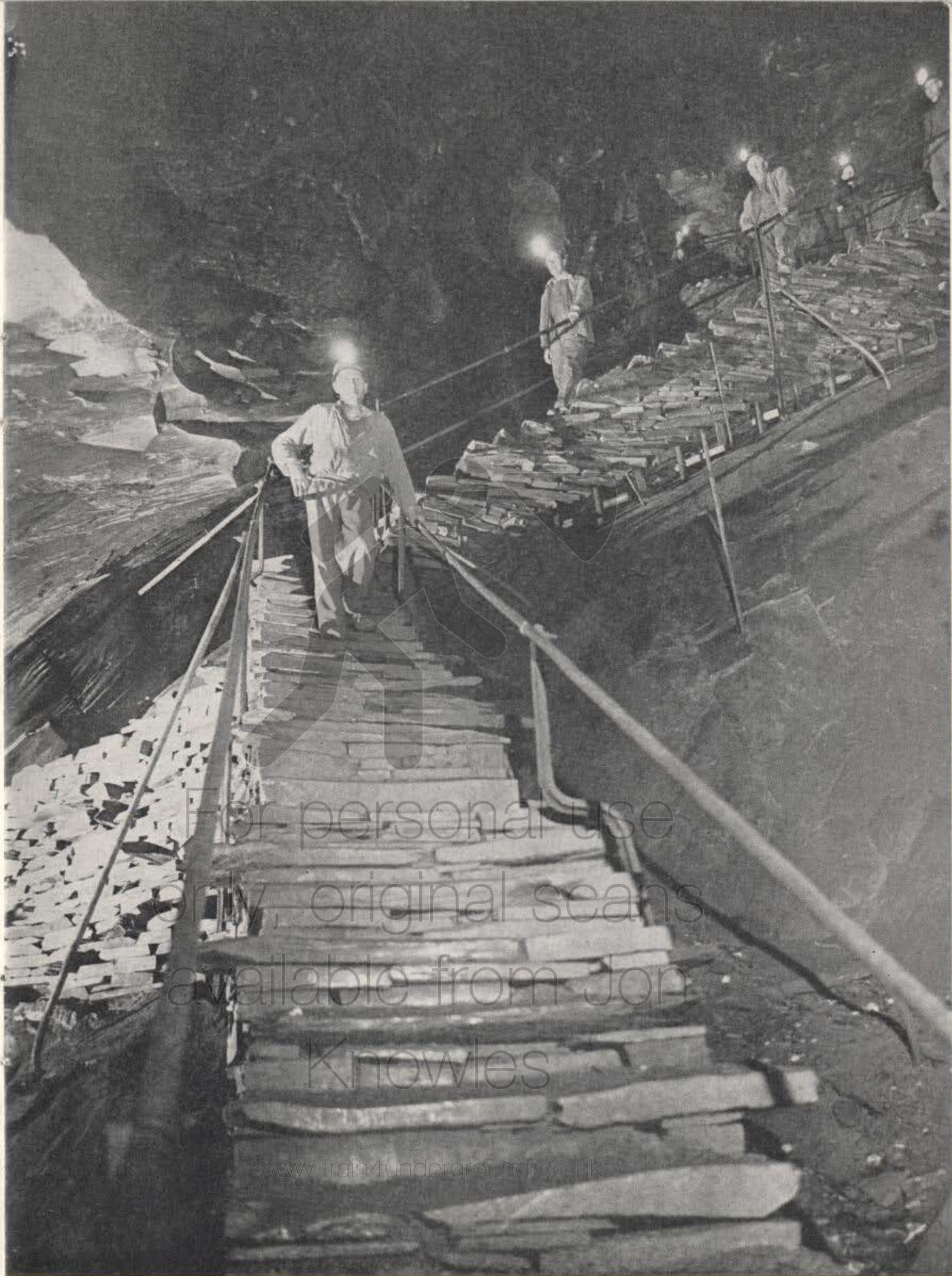
This hand-railed zig-zag stairway—"Grisia" to quarrymen—links K and L floors of the Oakeley mine. Built with slate slabs of course, it typifies other stairways connecting working levels away from the central inclines.
