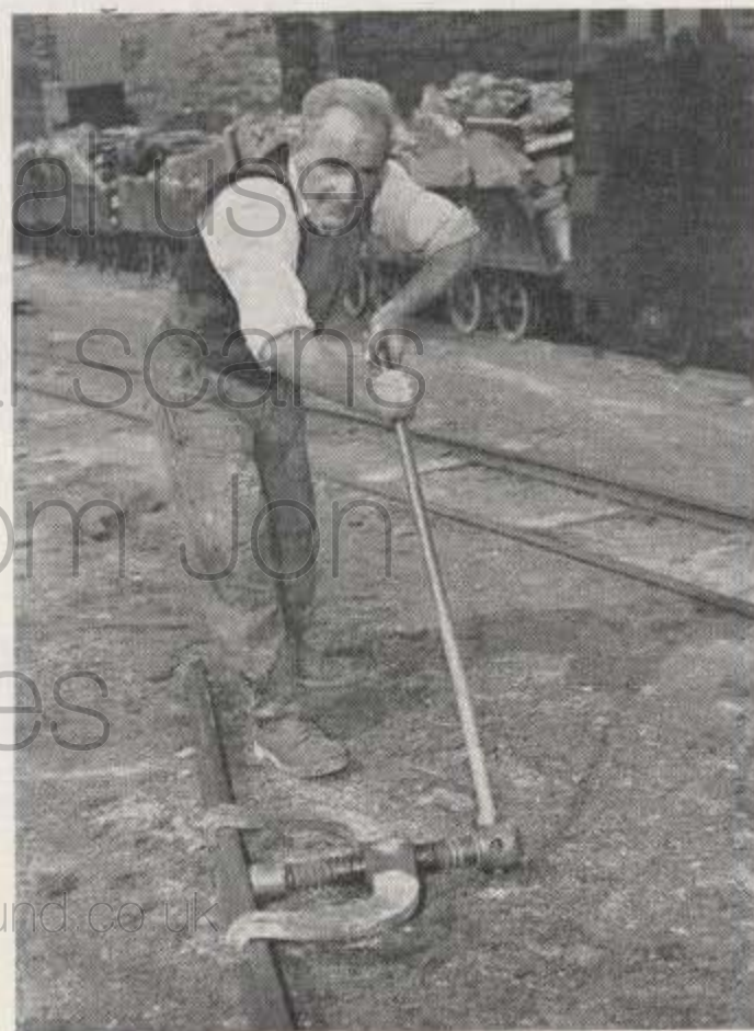
Platelayer William Llewelyn Owen demonstrates the use of the "Jim Crow," the piece of equipment employed for bending rails.
